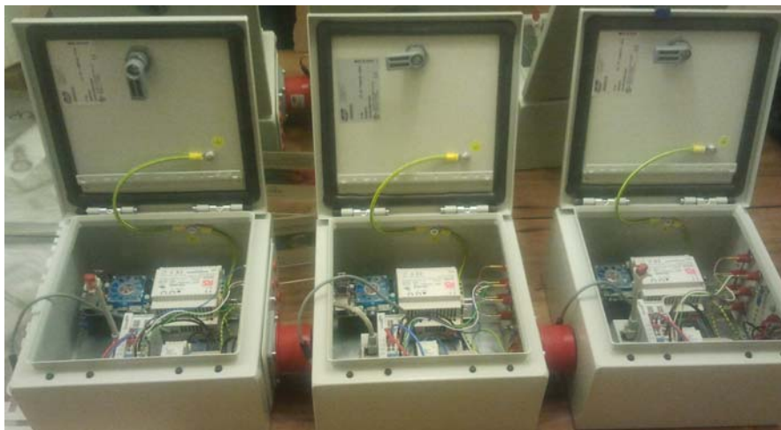
Figure 37: Hardware boxes to measure the main electrical machine connection
